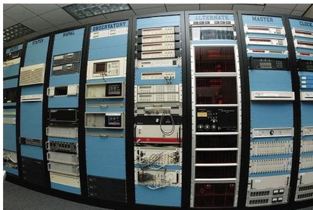
The U.S. Naval Observatory Alternate Master Clock at Schriever AFB (Colorado) is a Stratum 0 source for NTP
